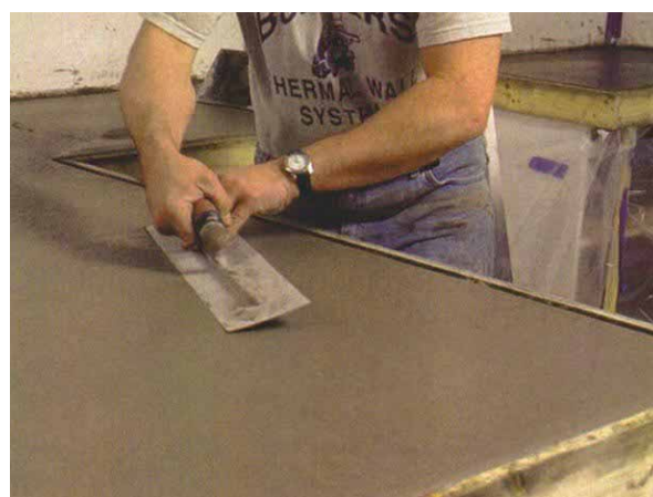
5. A steel trowel polishes the surface.
