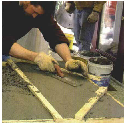
1. Pack the concrete into the forms.
