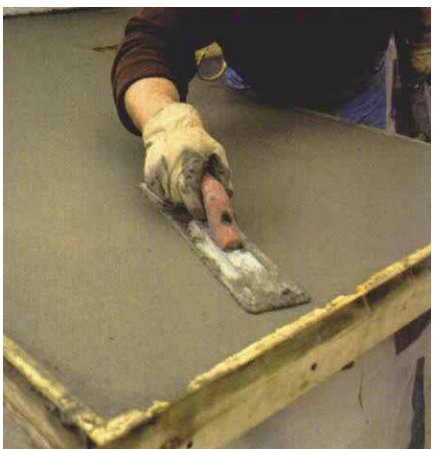
3. The mag float flattens the surface.
