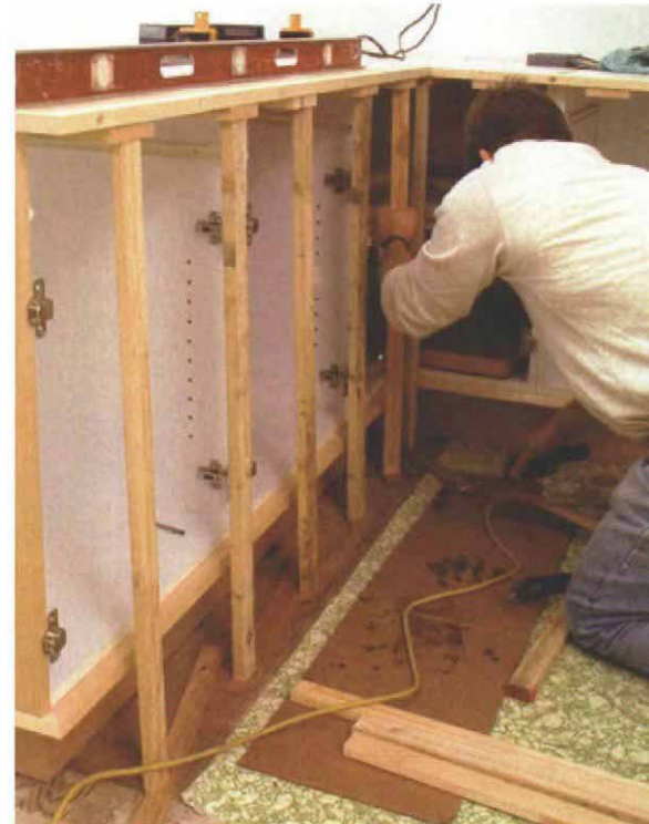
Add vertical supports. Beneath each brace, Mark Story wedges a 1x post. The bracing will prevent the forms at the overhang from flexing as the concrete is poured and troweled.
