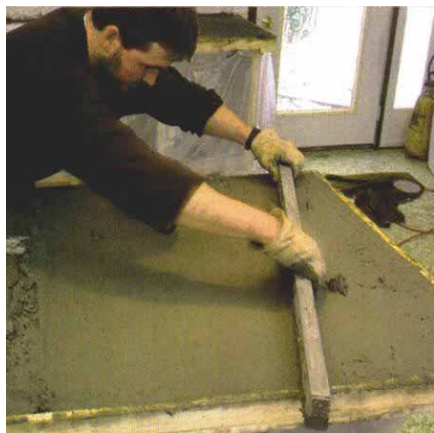
2. Remove the braces, and screed the top.
